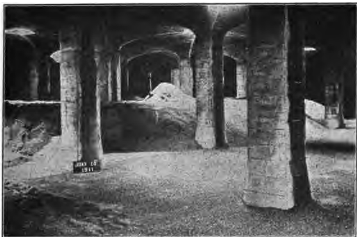
FIG. 43b.—A portion of the same filtration beds filled with sand ready for filtration.
